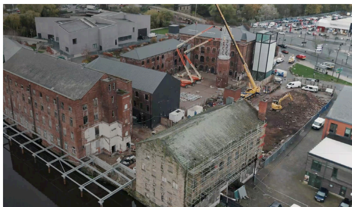
Rutland Mills development (Tileyard North)
