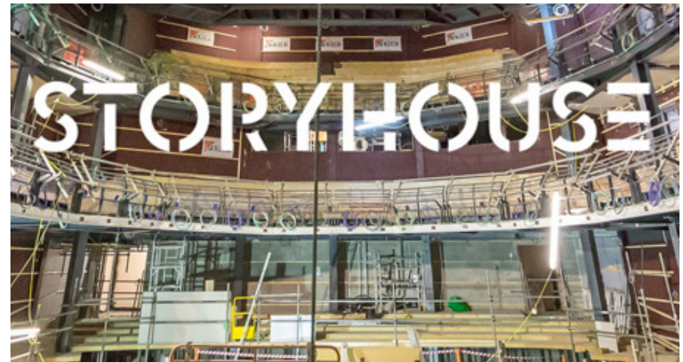
Picture 26. Chester Storyhouse construction
